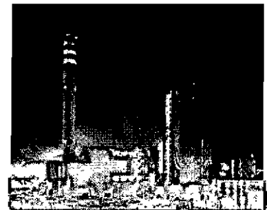
ELCHO Location: Chorzow, Poland Customer: EC Chorzow Elcho Sp. z o.o. Start-up Year: 2003 Capacity: 2 X 113 MWe Fuel: Bituminous Coal
